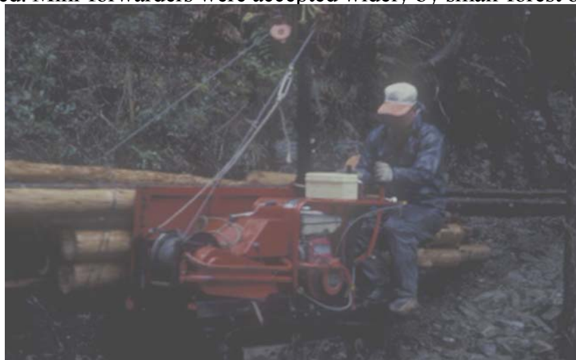
Figure 3. Mini-forwarder with rubber crawlers on an operation road 1.5 m in width (1984) [2]
